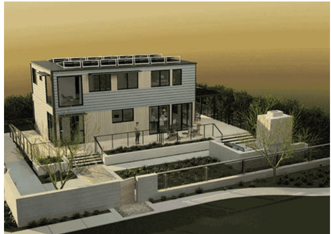
Figure 1: Now operating, this home in Southern California demonstrates practical implementation of a future residential energy system.
